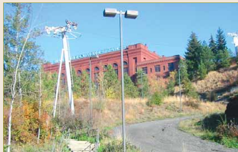
Fountains, public art and wayfinding signage will tell the story of the City's connection and history with the Spokane Falls.
