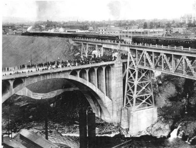
Figure 2: Spanning the bridge that spanned the falls. By 1912, the Union Pacific Railway bridge was constructed over the hydro station, the Monroe Street Bridge, and the falls, barely visible in the lower right corner. Note the extensive backfill placed to accommodate the rail grade. ( Eastern Washington State Historic Society )
